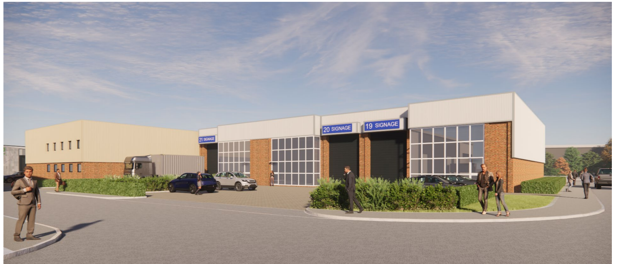
▲ Zone 1, Units 19-21 - Existing
