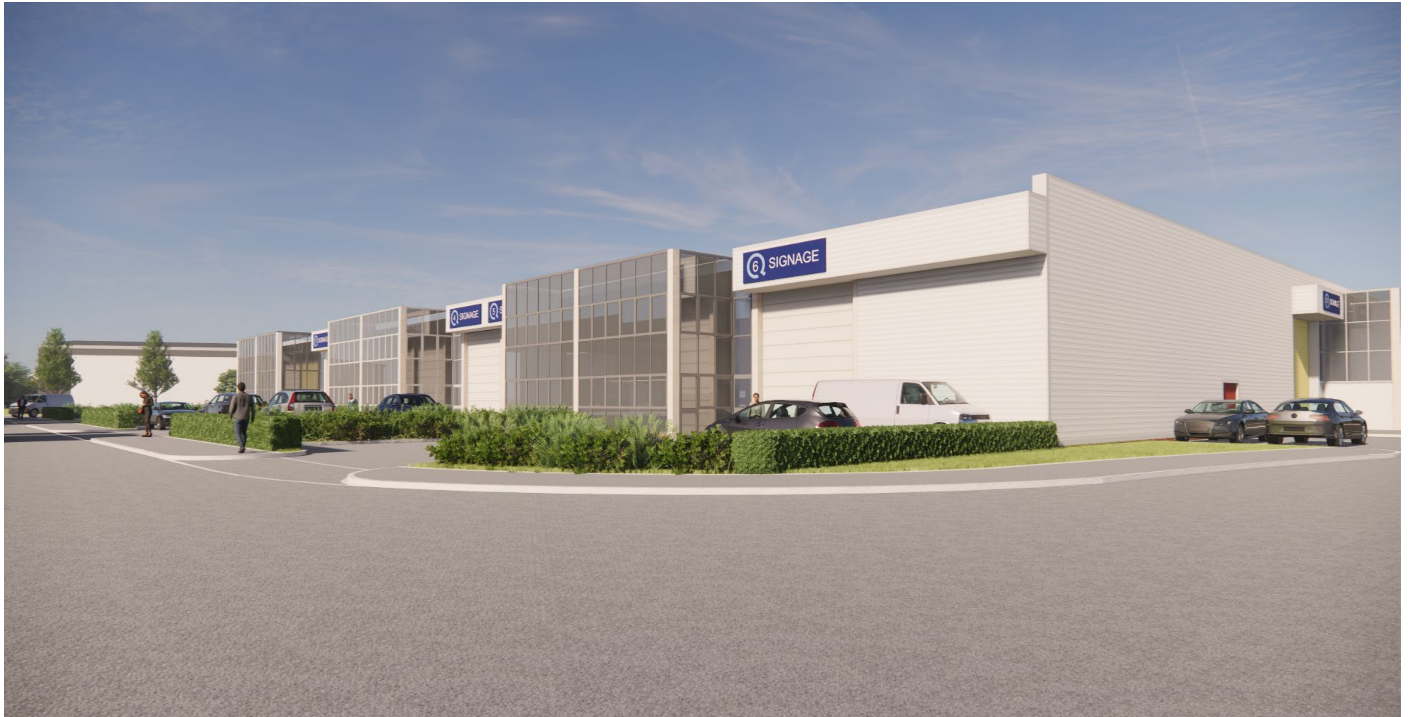
▲ Zone 2, Units 1-6 - Existing
